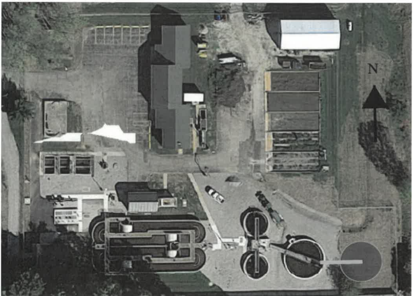
Figure 2.2 Aerial Photograph of Wastewater Treatment Plant
